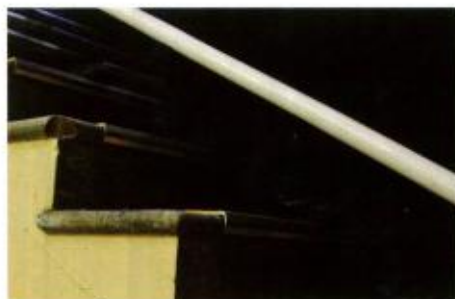
Above: Bright yellow nosings have made changeovers somewhat more safer.
